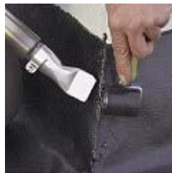
Welding bitumen
